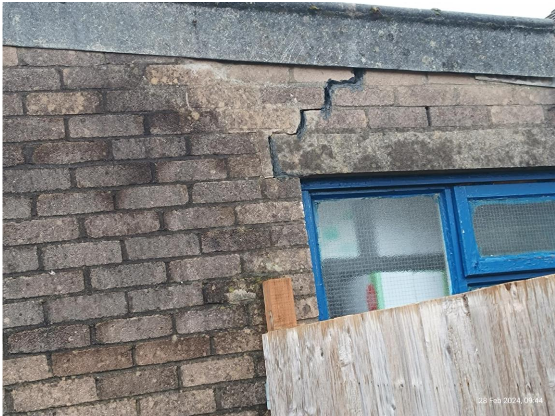
Stepped cracking to brickwork at side of outbuilding
