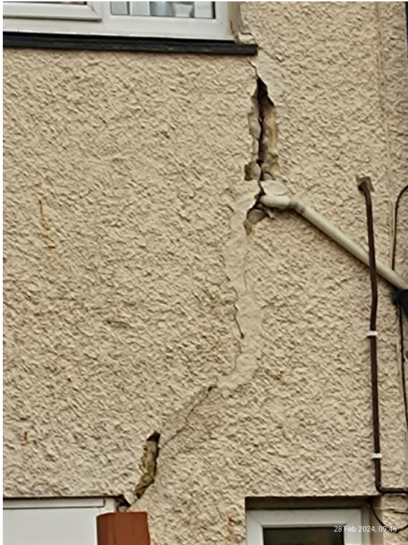
Cracking to external envelope
