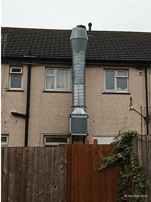
Extraction unit from Chinese takeaway
