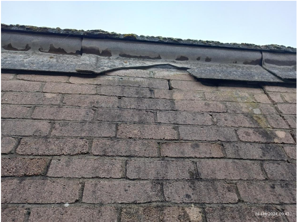
Damaged asbestos roof sheets to front elevation of outbuildings
