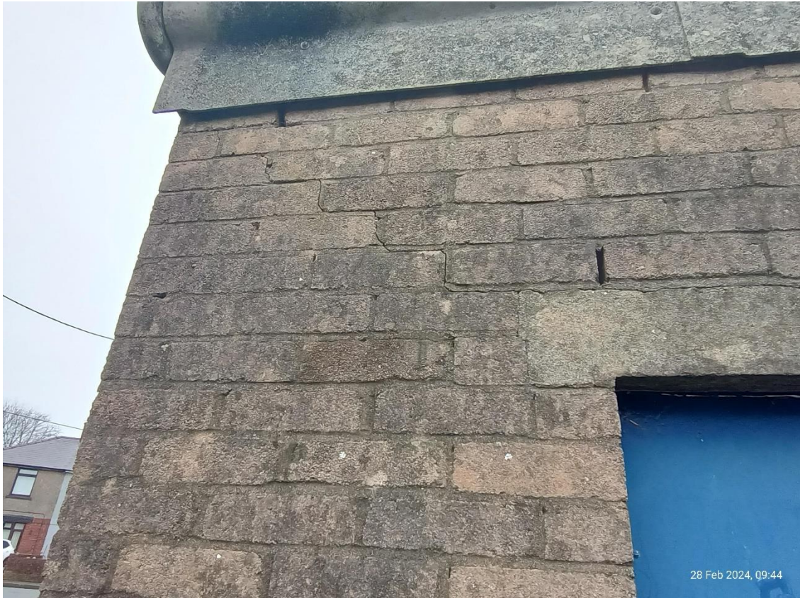
Stepped cracking to outbuildings
