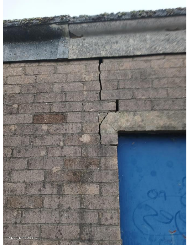
Cracking to brickwork on outbuildings
