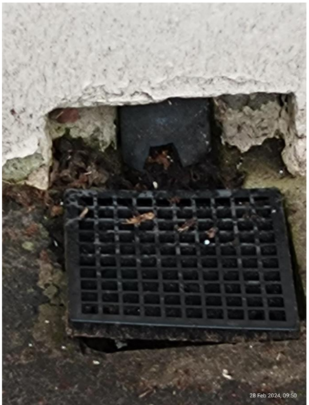
Downpipes exiting building fabric to rainwater gulley
