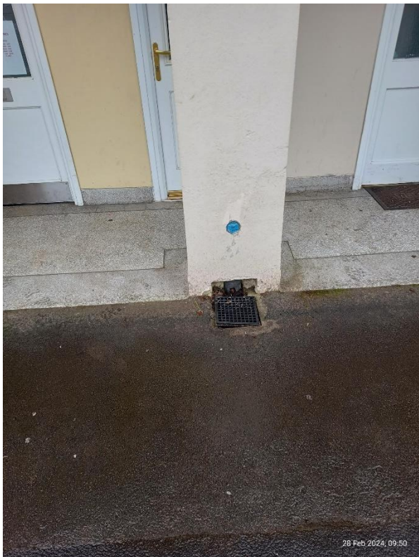
Downpipes exiting building fabric to rainwater gulley
