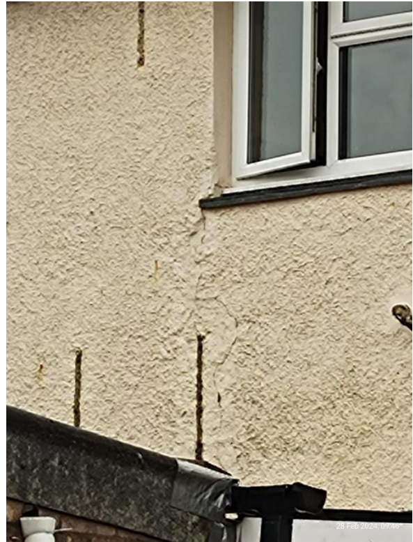
Cracking to external envelope
