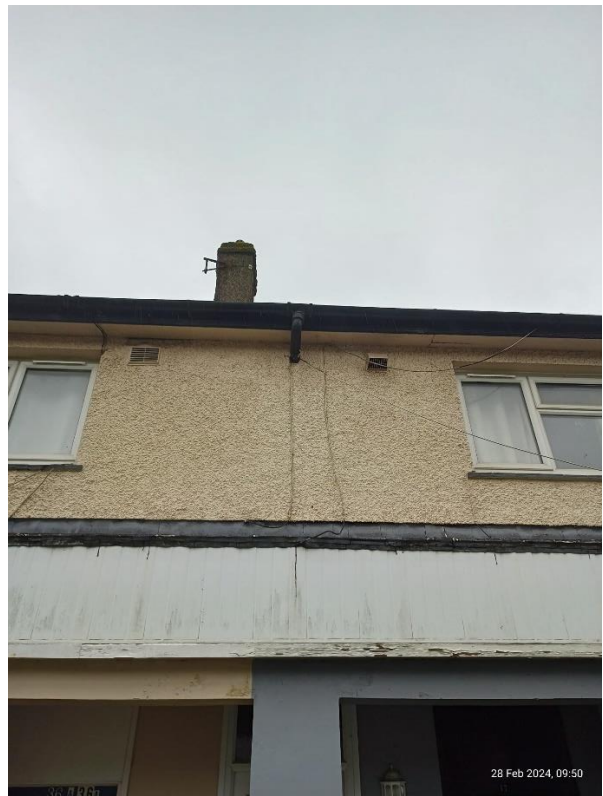
Downpipes built into external walls to front
