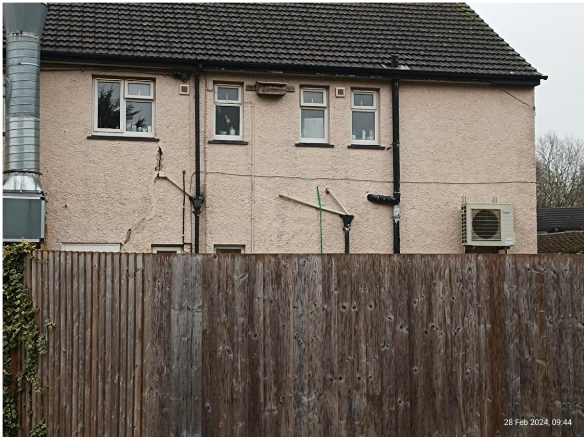
Soil vent pipes extending through soffit and roof at eaves level
