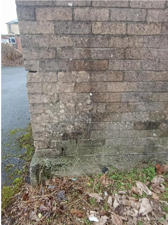
Cracking to brickwork on outbuildings
