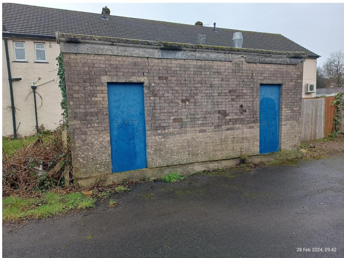
Cracking to brickwork to front of outbuildings
